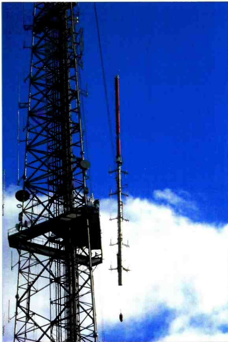
WRC, Washington, DC, chose to stack its NTSC antenna at 587 feet and its digital antenna at 637 feet. Shown are the antennas being raised into position.
